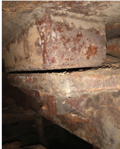
Side bearing clearance
